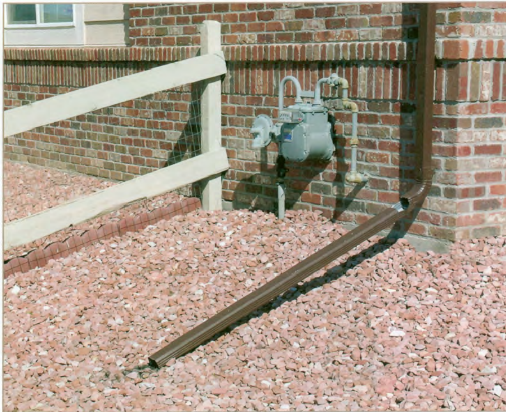
A gravel-covered runoff slope with a downspout extension to carry water away from the foundation.
