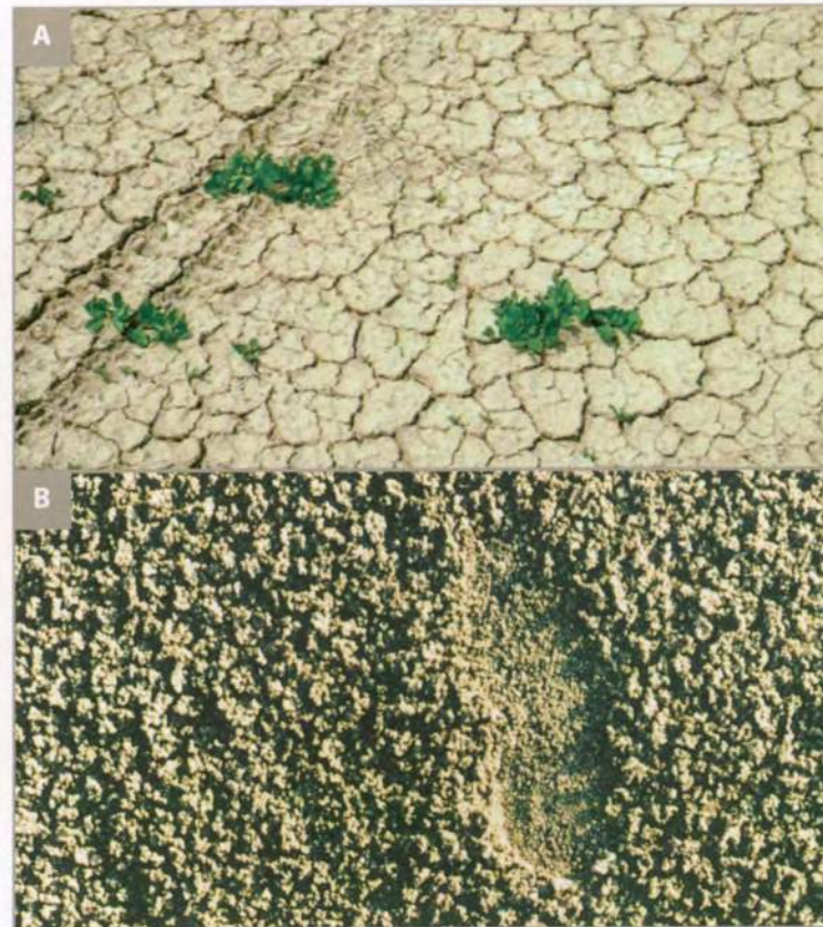
Evidence of swelling soil at the ground surface. A) Small-scale desiccation cracks, with tire tracks for scale. B) “Popcorn” texture, with footprint for scale.
