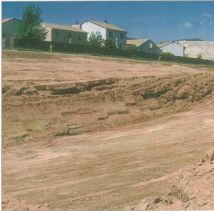
An overexcavation and fill replacement construction operation.
