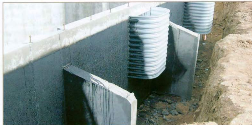
Concrete buttress installed along the outside of a foundation wall.
